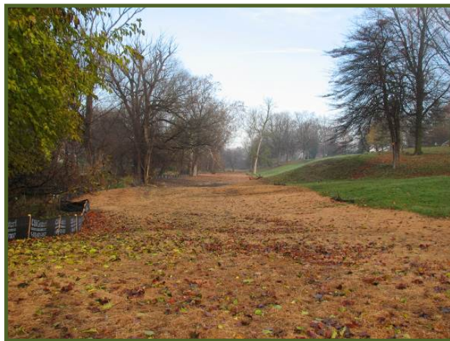
Silt fence installed at Lola Valley Park November 15, 2011
